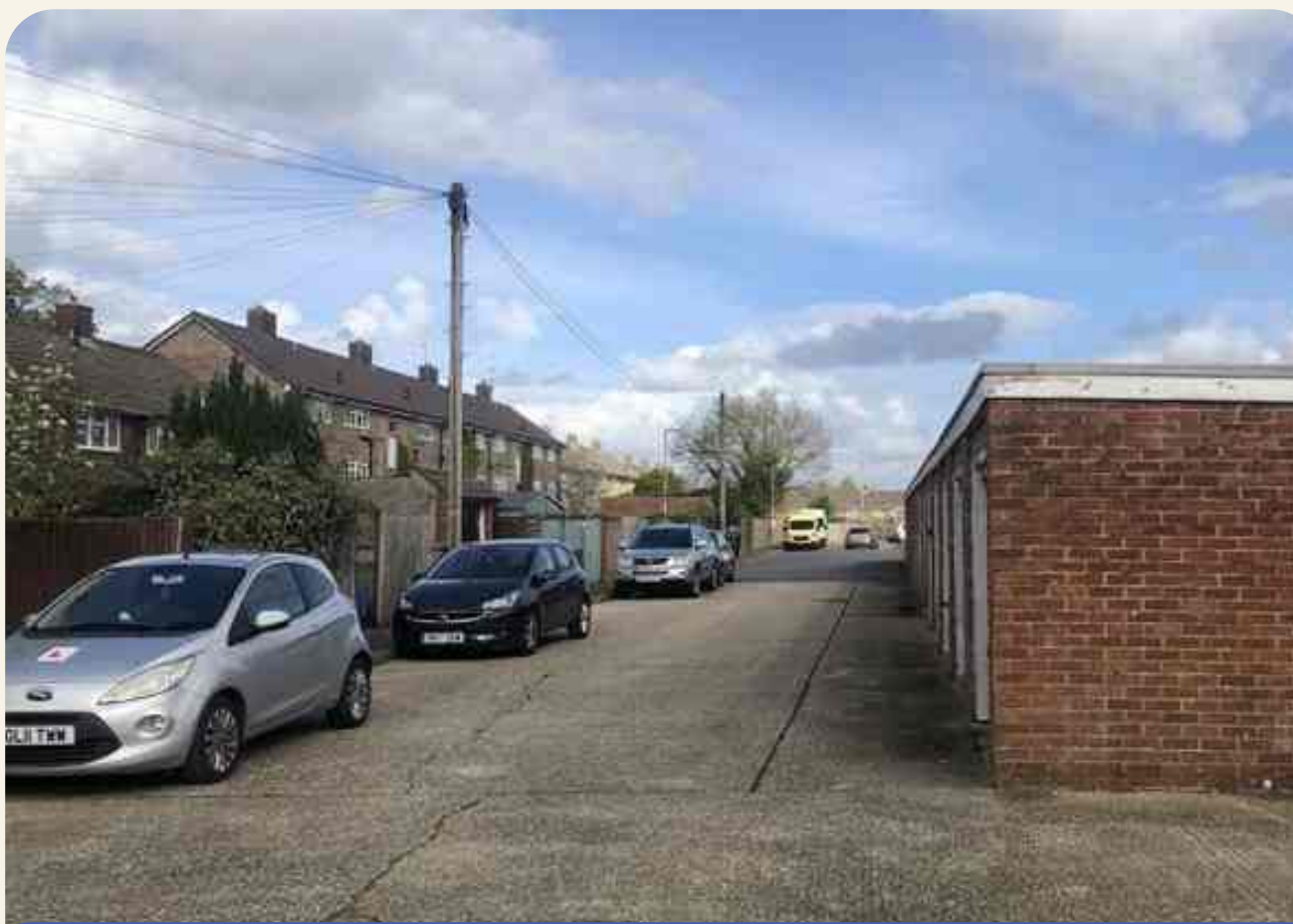
Existing garages and parking area, southwest corner of site
