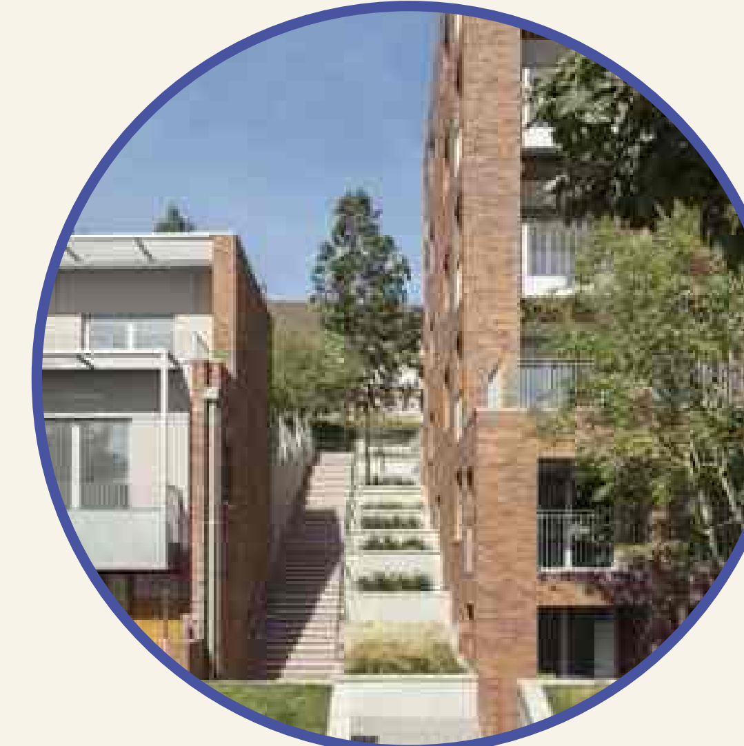
Different building heights and shapes
