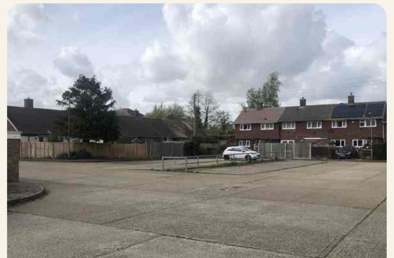
Existing parking court to north of the site
