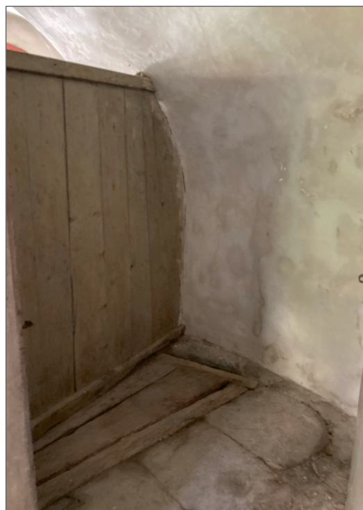
Foto 12 Raum 3 Erdgeschoss | Vano 3 piano terra
