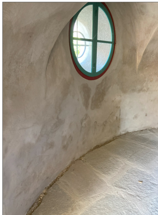
Foto 10 Raum 1 Erdgeschoss | Vano 1 piano terra
