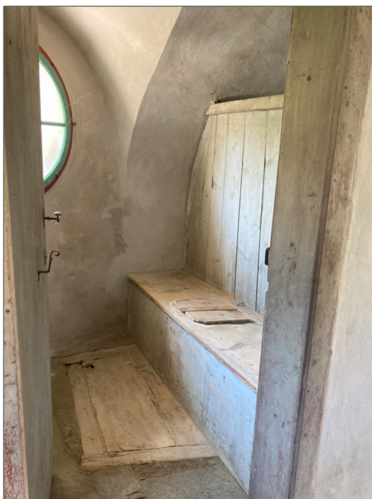
Foto 11 Raum 2 Erdgeschoss | Vano 2 piano terra
