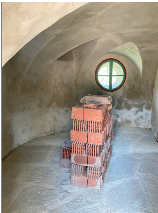
Foto 09 Raum 1 Erdgeschoss | Vano 1 piano terra
