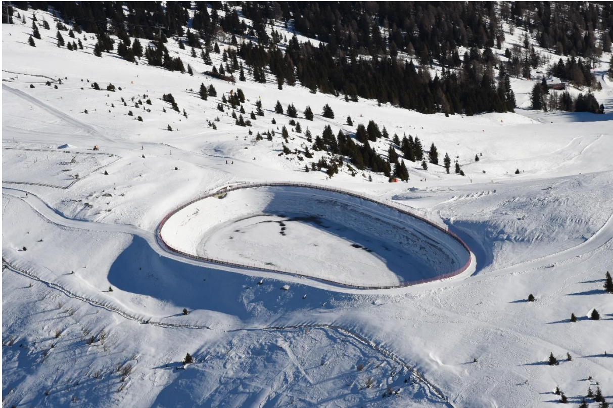
Beschneigungsbecken „Hinterberg“. Bacino di innevamento “Hinterberg“. “Hinterberg” storage basin for technical snowmaking.
