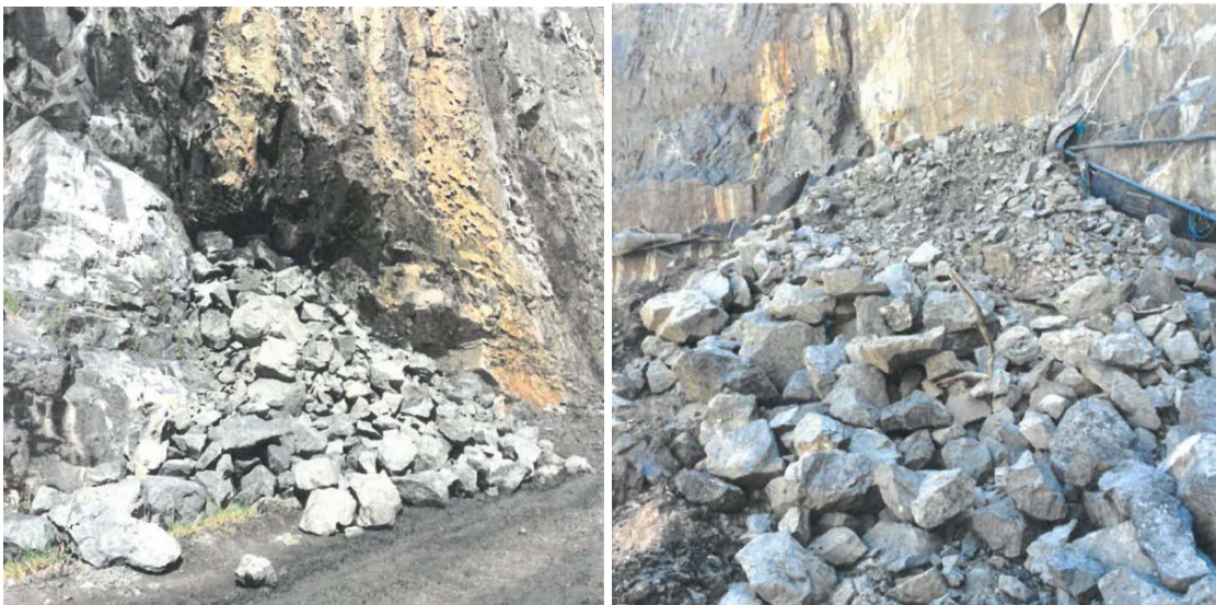
Figure 6 Photographs of the sealing of the underground portal
