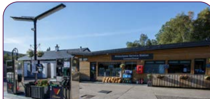
KINLOCHEWE SERVICE STATION, WESTER ROSS, HIGHLAND
