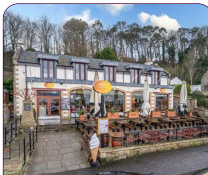
RAILBRIDGE BISTRO, SOUTH QUEENSFERRY
