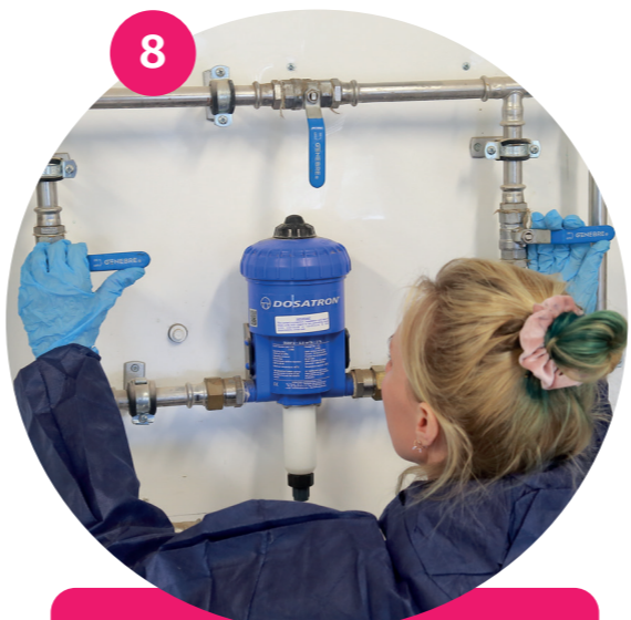
8 Adjust the dosing mechanism to the appropriate dose rate and switch on
