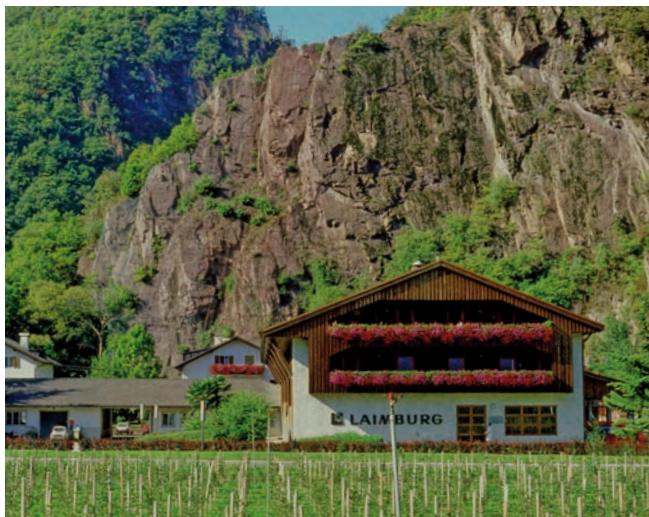
The stable, later converted into administrative offices
