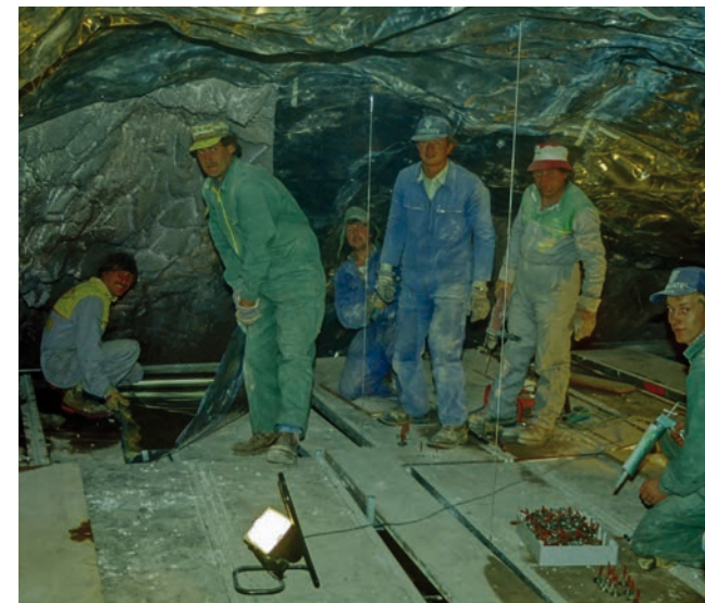
Construction of the Rock Cellar
