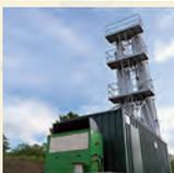
Biogas is produced, a gas scrubber enables injection into the mains gas grid
