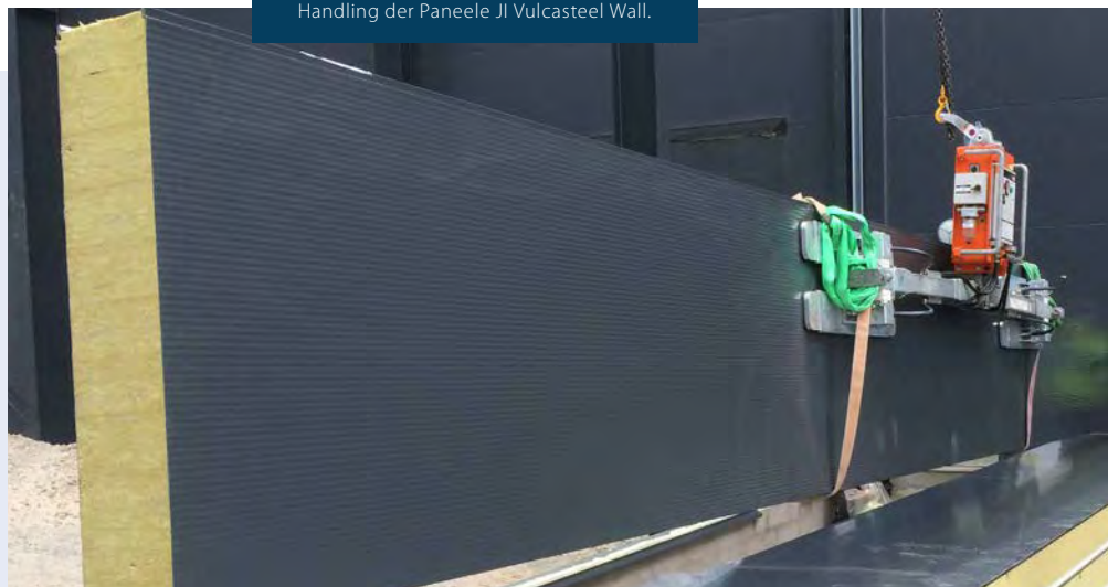
Handling der Paneele JI Vulcasteel Wall.
