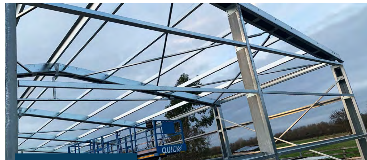
Raw structure of the Kit building skeleton.
