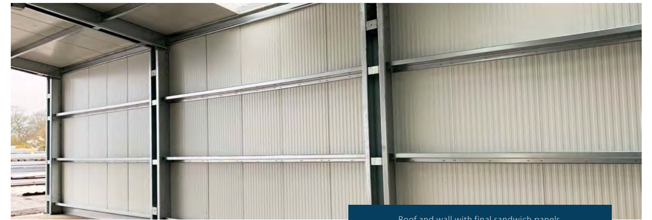
Roof and wall with final sandwich panels.
