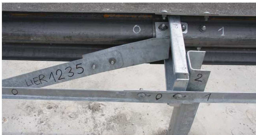
↑ Fixation tirant / Brace fixing / Attacco tirante
