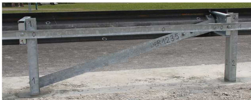
↑ Tirant entre les supports n°1 et 2 / Brace between posts nrs. 1 and 2 / Tirante tra i paletti n°1 e 2 ↓
