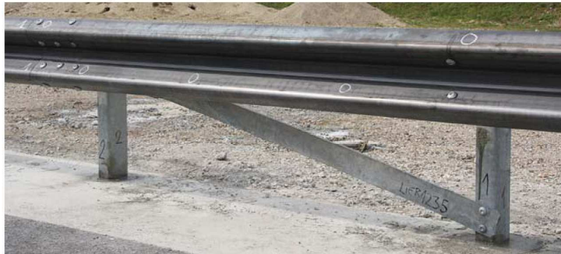
↑ Tirant entre les supports n°1 et 2 / Brace between posts nrs. 1 and 2 / Tirante tra i paletti n°1 e 2 ↓
