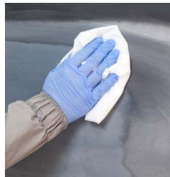
Clean the repair area
