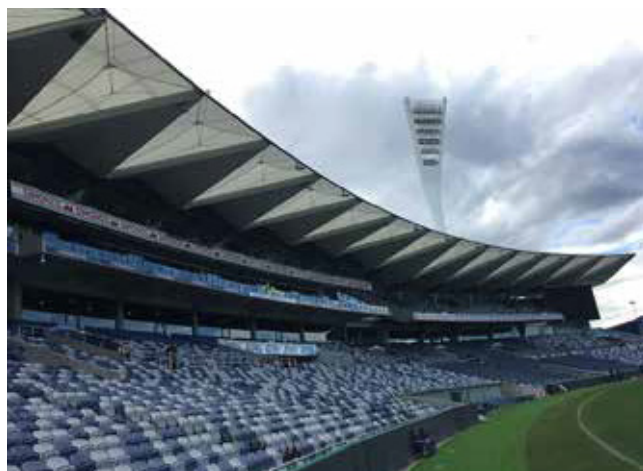
Simonds Stadium Stage 4 – grandstand from inside the arena
