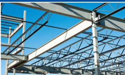
Structural steel and support systems
