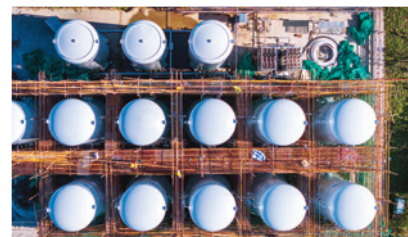
Water and wastewater systems
