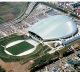
▲ At the 2002 World Cup, held in Japan and South Korea, the grass at the Sapporo Dome was grown away from the stadium and then moved as an entire pitch into the arena on a cushion of air.
