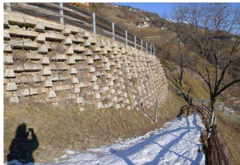
Betonkraierwand – muro cellulare in cemento
