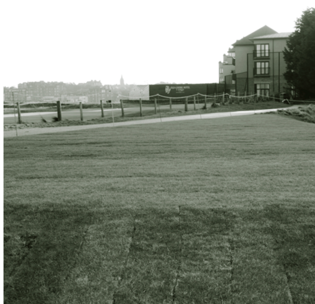
Construction of a new championship tee on the Old Course.
