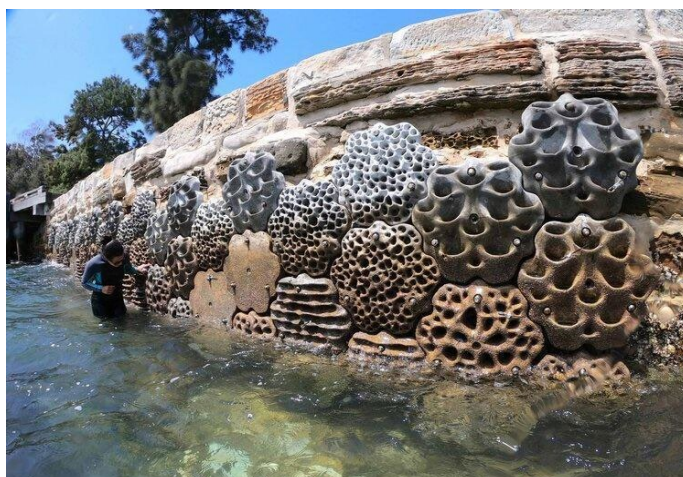
Figure A.4 An example of a 3D printed eco-seawall in Sydney (Living Seawalls, 2021)
