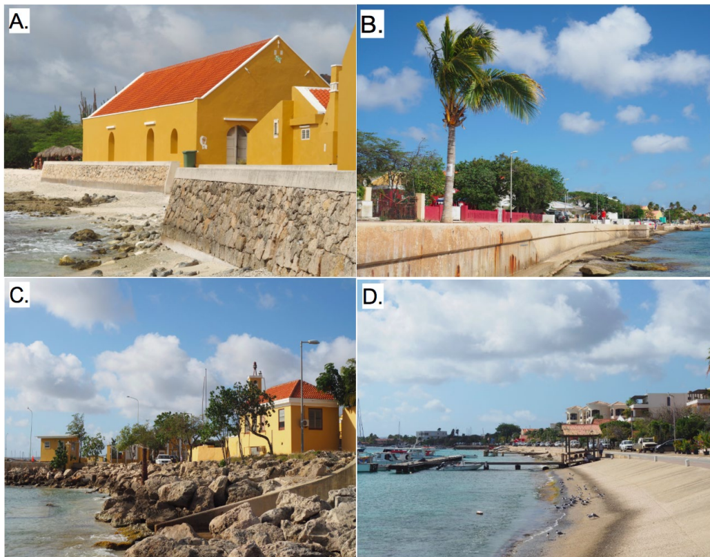
Figure 3 Example of grey coastal adaptation in Bonaire: A) traditional stone seawall, Boca Slagbaai, B) boulevard, Kralendijk, C) boulder revetment, Kralendijk D) smooth concrete revetment, Kralendijk (photos: author)
