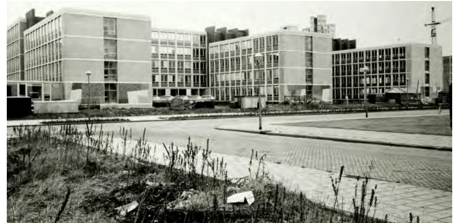
Back of the W & N building from A.J. Ernststraat (1969) (Note: the 5 th and 6 th floors came later)
