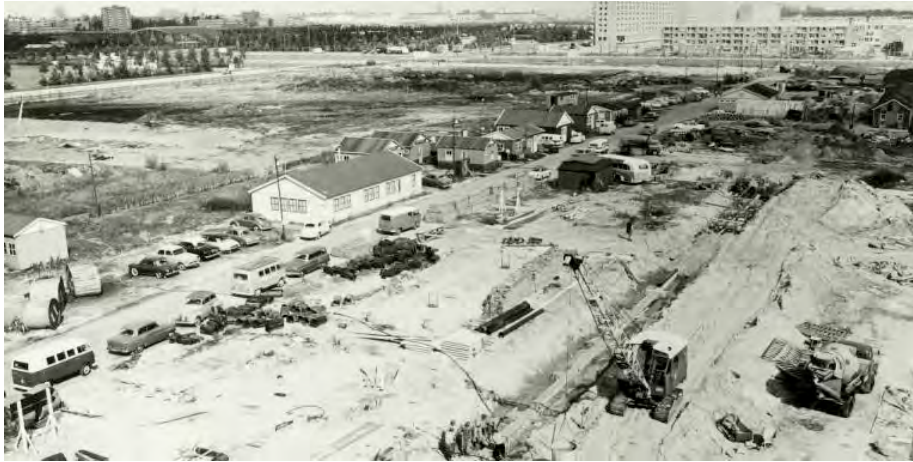
Start of construction of the W & N building (1965)
