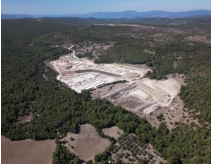
The Vastria CCAC under construction 64
