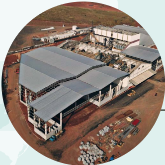
Warehouse and plant under construction in Varginha, Brazil
