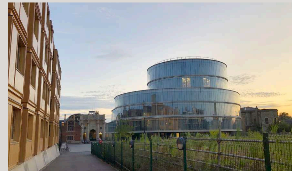
3. View looking southwest along Somerville College towards Blavatnik School of Government
