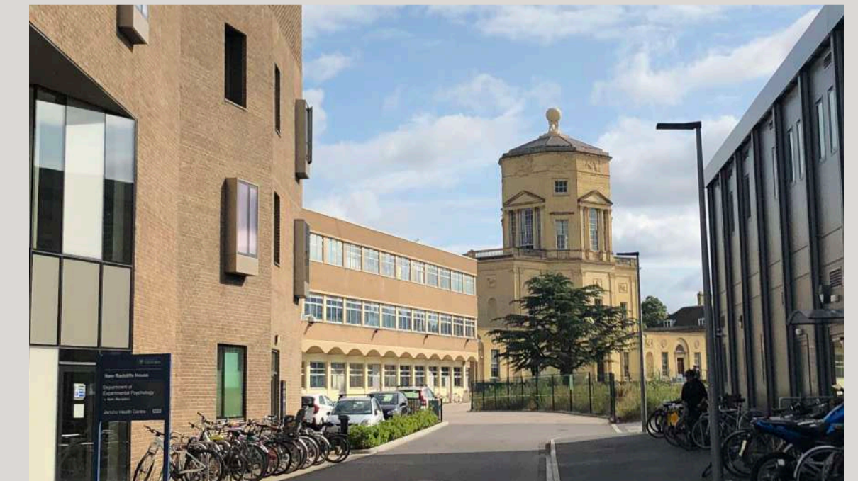
4. View of the site along the Harkness Building looking North East
