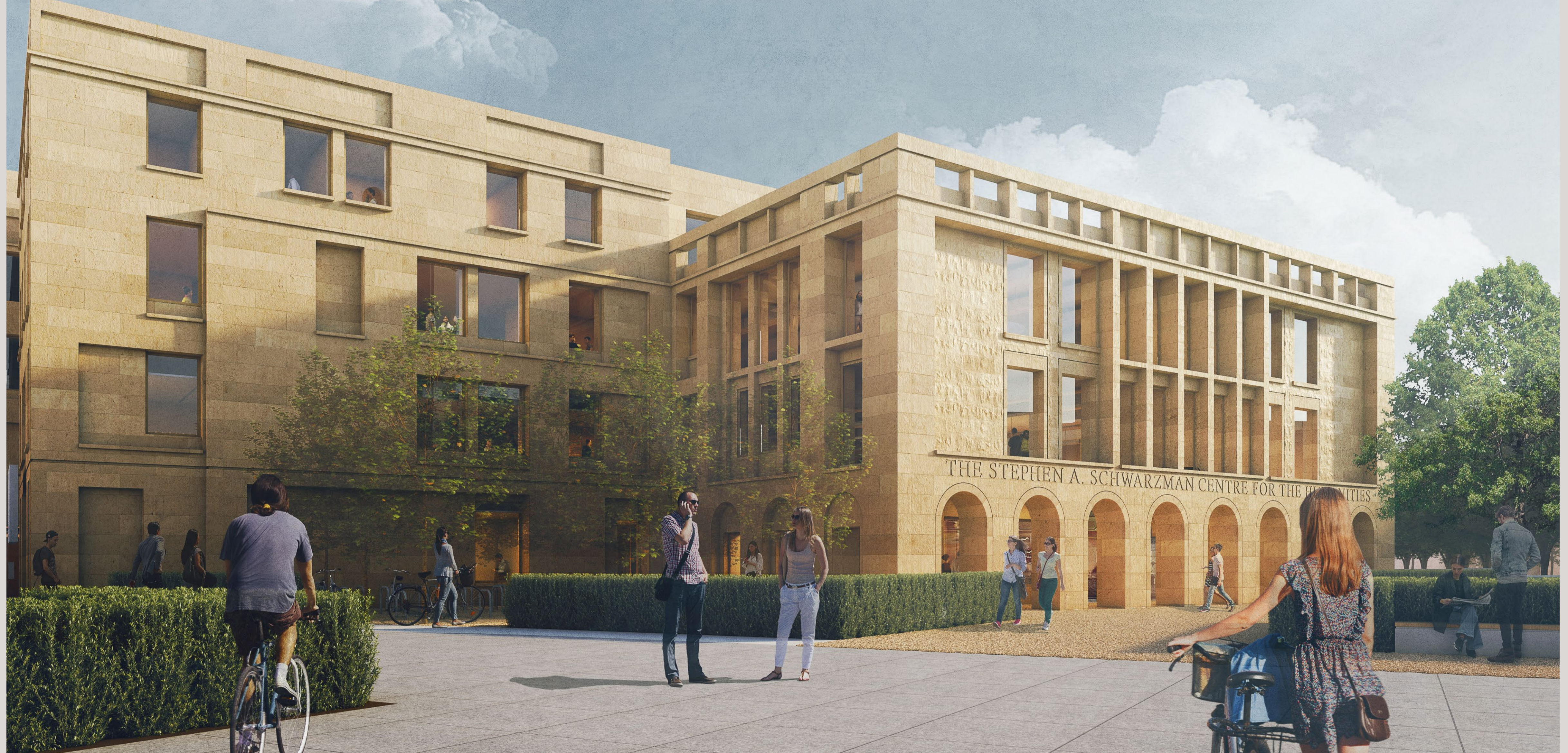
View of the Northern Entrance
