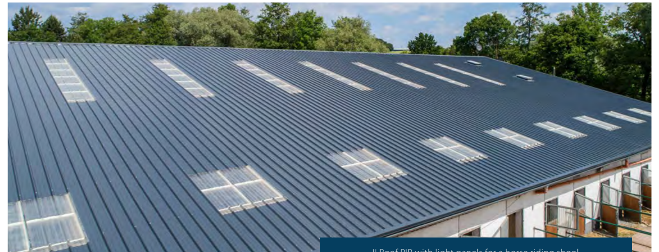
JI Roof PIR with light panels for a horse riding school.
