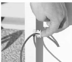
① Position grounding clip with electrical cable inserted in it and the bottom of the part outside the frame
