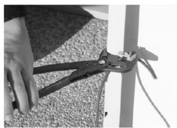
② Place the plier by gripping the clip with the external jaw and internal jaw set on external face of the module frame
