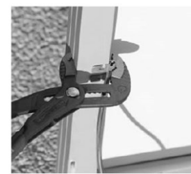
③ Grip up to the stops of the clip are against the frame
