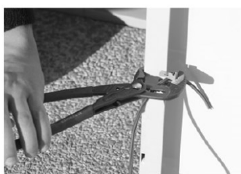
2 Place the plier by gripping the clip with the external jaw and internal jaw set on external face of the module frame
