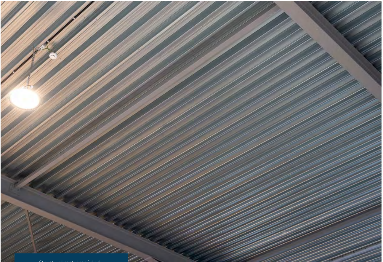
Perforated inner sheet for acoustic performance.
