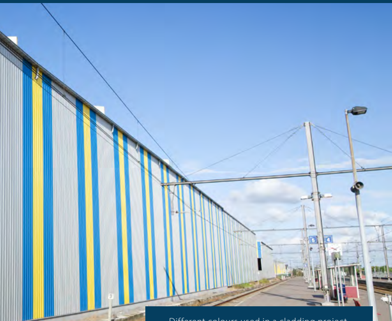
Different colours used in a cladding project.
