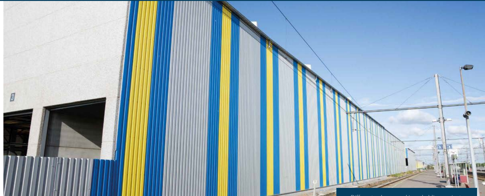
Different colours used in a cladding project.
