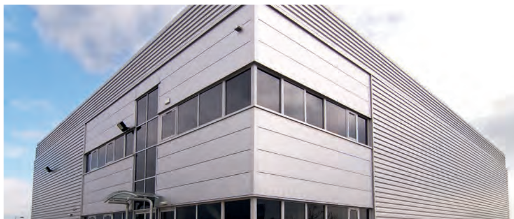
JI Wall 1000SF PIR in an industrial application.
