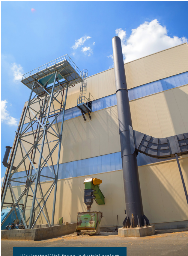
Jl Vulcasteel Wall for an industrial project.
