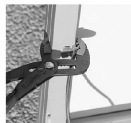
③ Grip up to the stops of the clip are against the frame
