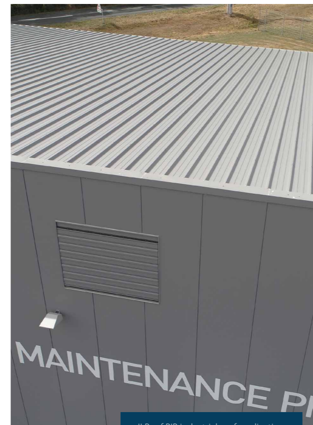
JI Roof PIR industrial roof application.
