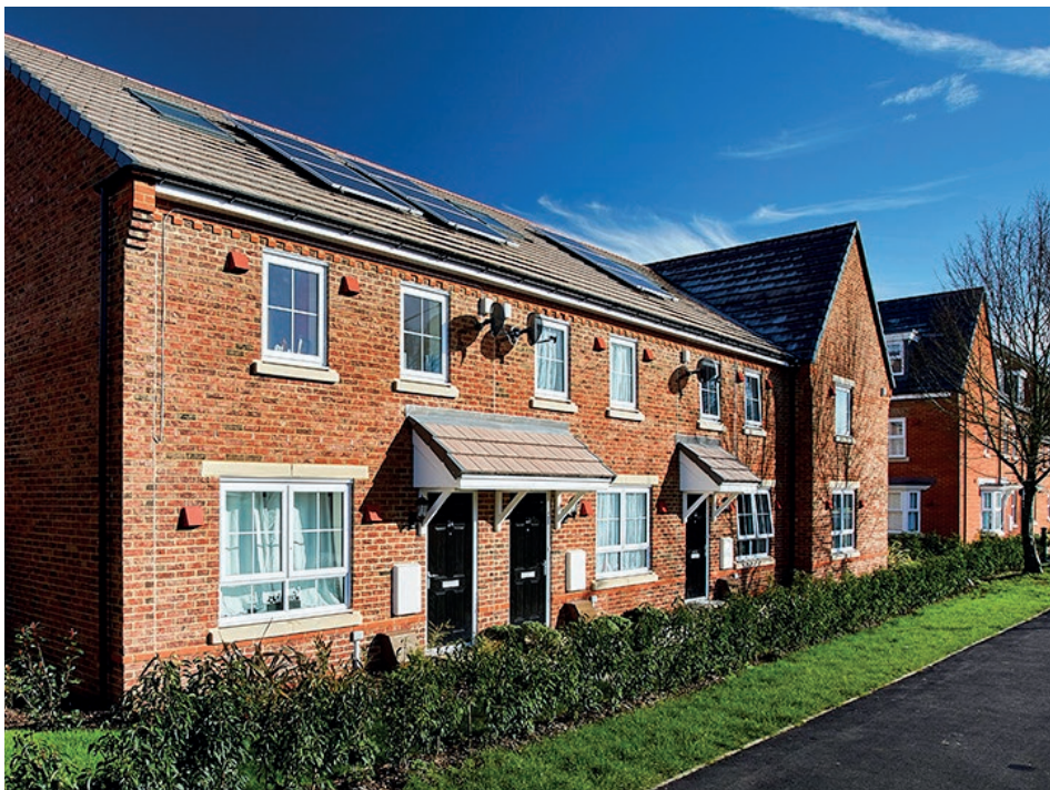
A joint venture with David Wilson Homes has transformed Kersey Crescent, Newbury, providing homes for social rent and shared ownership.
