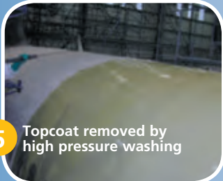
4 Topcoat further attacked and removed by stripper
