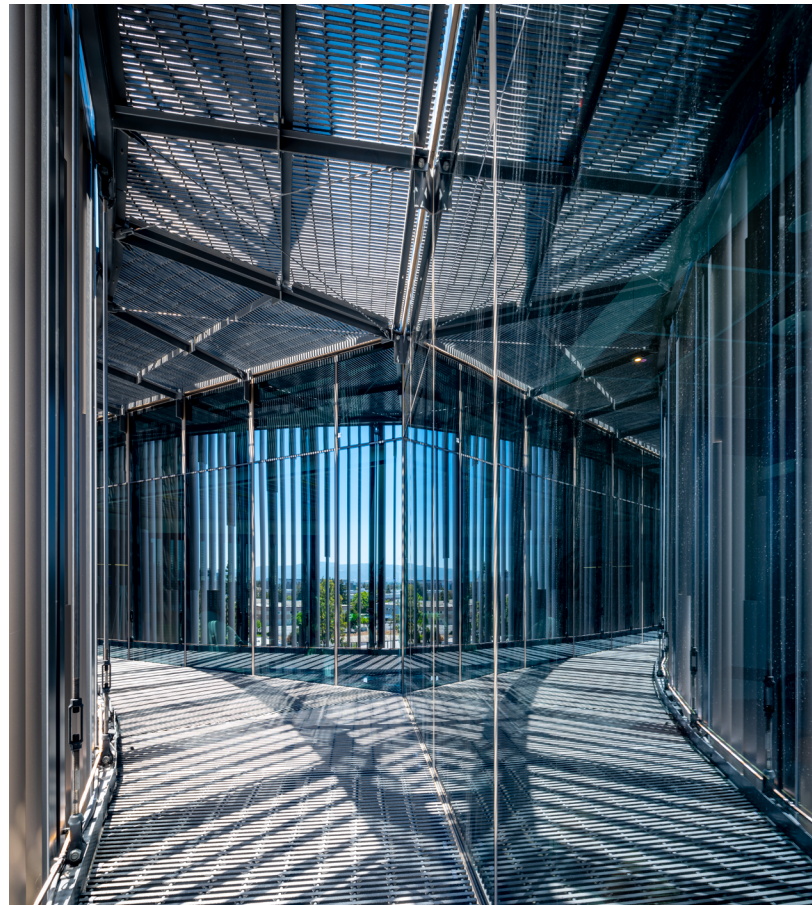
VikingSteel fabricated and installed the catwalk that connected the louvers to the curtain wall, an integral part of the facade assembly. R&B Protective Coatings finished it with the non-metallic zombie black coating.
