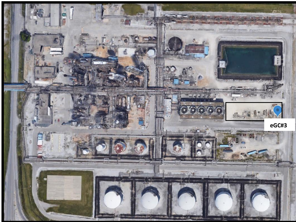
Figure 2: Area fork truck was operating in relation to the whole INEOS Styrolution Sarnia Site.
